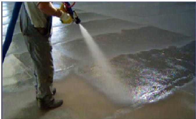
Low pressure spray application
