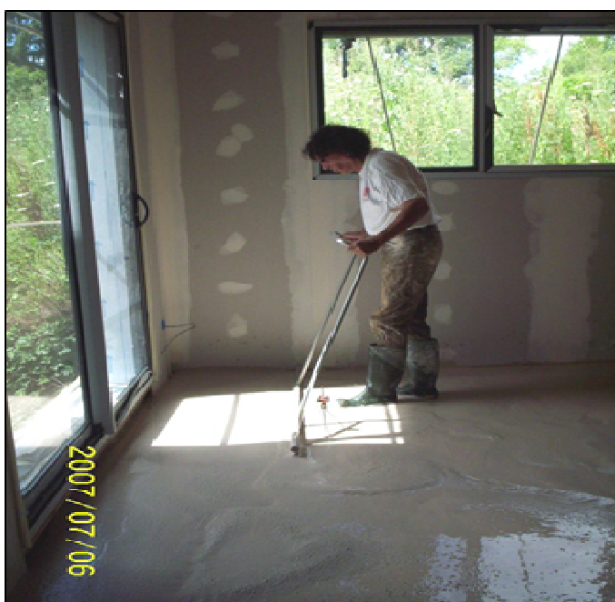
Execution of anhydrite screed over primer
