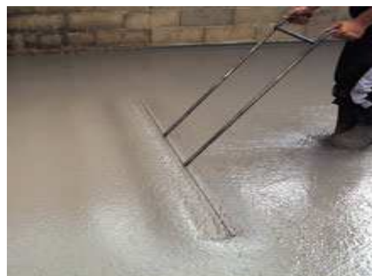
Figure 1: Equalisation of a screed after execution with EURO NIV HP
